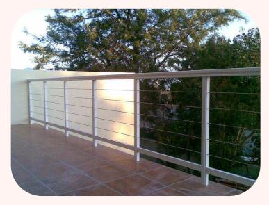
The New York stainless steel cable balustrade uses only marine grade 7x19-316 stainless steel cable. The 316 SS cable will not rust or corrode and is therefore maintenance free. Gaps between cables do not exceed 100 mm and complies with all regulations relating to balustrades.
