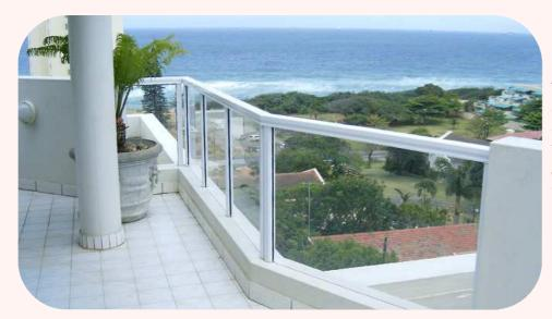
The clean lines of the New York glass and aluminium balustrades compliment the aesthetics of modern home designs. Only the highest quality 5 mm Toughened safety glass is used in accordance with SABS 0400 - Part D. All installations make use of the highest quality injection mortar and fixing methods. Tinted or sandblasted glass can be fitted on request.
