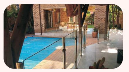
The Glass Pressure Brackets are attached to the stanchions and clamp the glass panels in place. The stanchions for this balustrade can be flange fixed or side-mounted.
